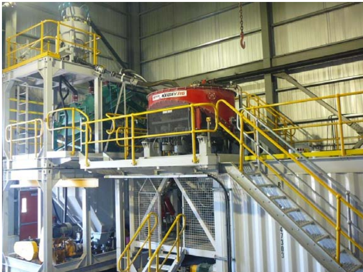
Modular Plant constructed at Niobec
